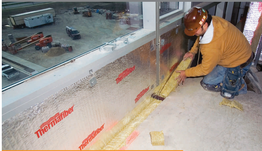
Thermafiber Safing is compression fitted between FireSpan insulation and the concrete slab edge to create a perimeter fire containment system.
